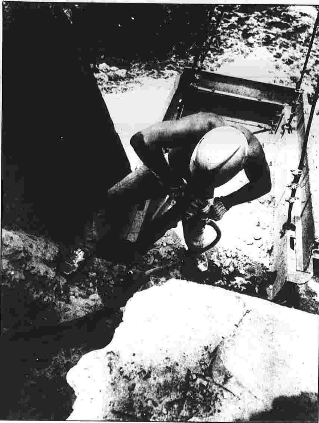
DAM WORK — Tom Dubois, of Danielson, uses a jackhammer to break concrete around the Union Pond dam as
